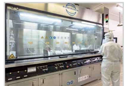
New stainless steel plant to process products using organic solvents
